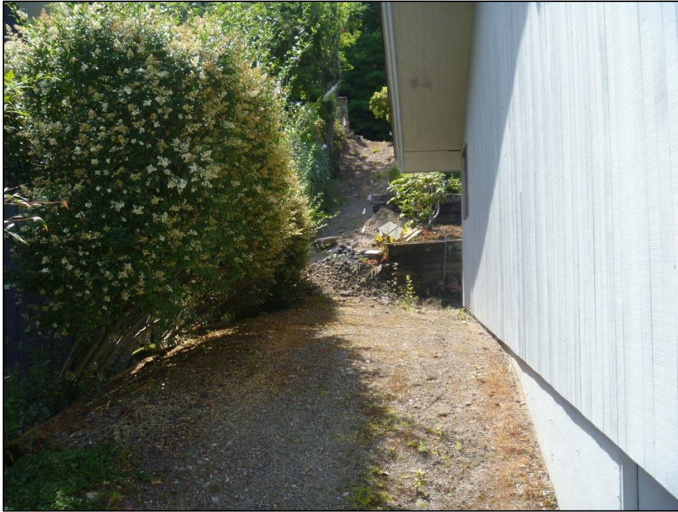
Figure 5: Watercourse A buffer reduction area (located within house footprint), facing west (6/18/2018).
